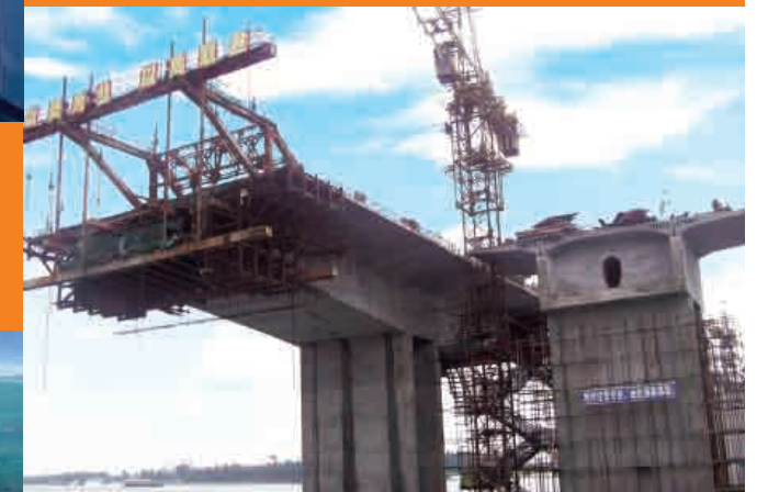
Construction of Phase II of the Western Delta Route linking Shunde to Zhongshan (Under Construction)
