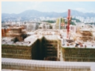
Construction of St. Teresa Hospital is in progress
