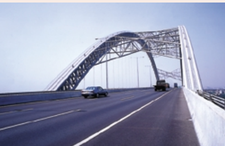
The grand construction work of Ya Ji Sha Bridge
