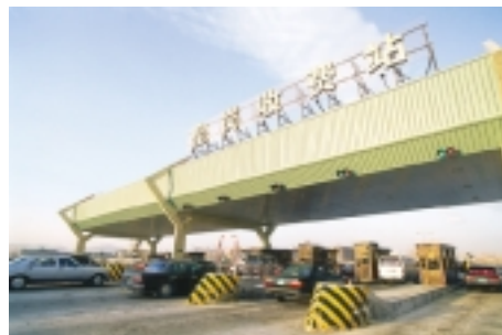
Toll station at Huanggang, GSZ East
