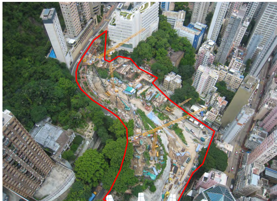
HCII Site – Site formation work in progress
